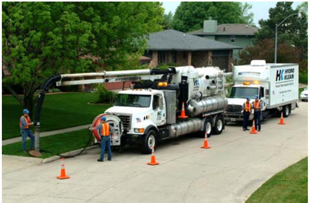
HK Jet/Vacuuming and Video Inspection Crews
