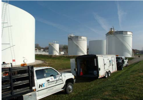
Overview of a Tank Farm
