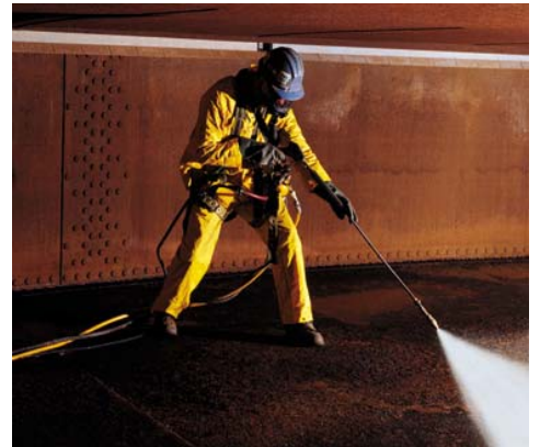
HK Sr. Service Technician, Shawn VonStein, Power-washing a Tank
